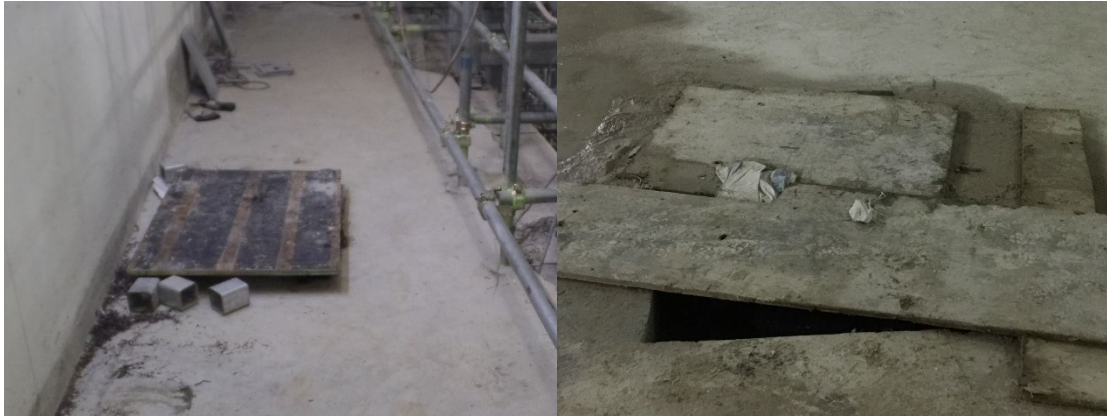
Figure 22 Floor openings with temporary covers such as planks and timber boards
