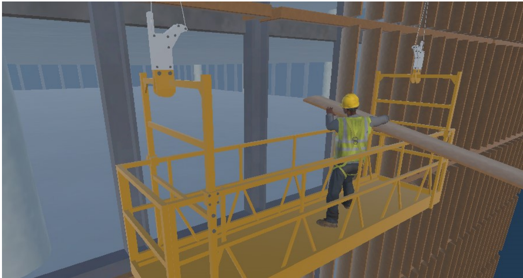
Figure 20 Long protruding vertical fins that need to be installed manually by workers on a gondola
