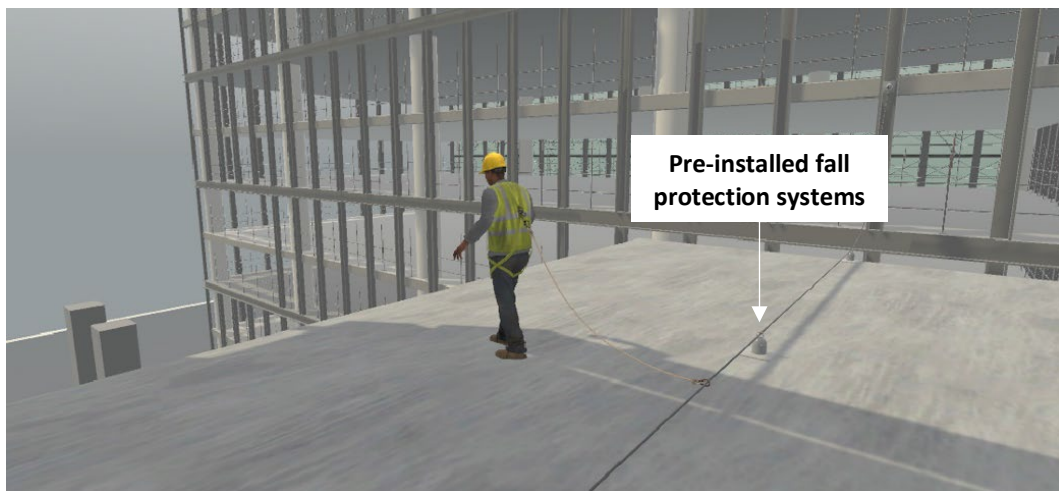
Figure 14 Design for fall protection systems that are pre-installed before link bridge is lifted into place
